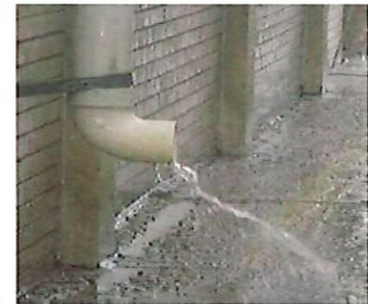
This downspout connects to the roof gutter.
